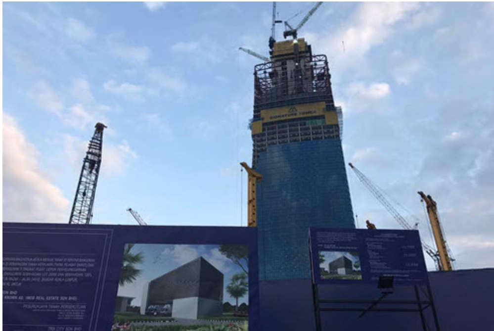
Construction is progressing on the 106-story Signature Tower skyscraper in Kuala Lumpur.
